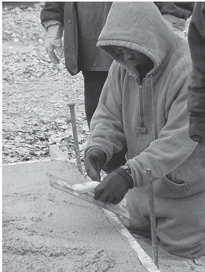
A TrANS student learns how to lay cement.
